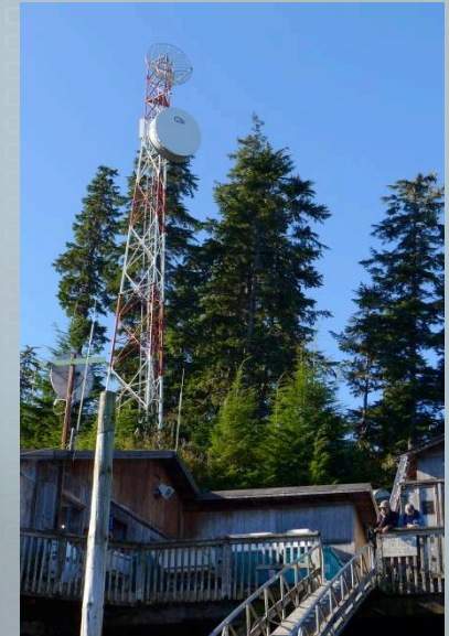
Port Protection: Microwave tower
